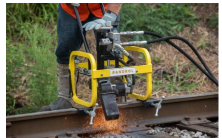
Grinding with head wash grinder.
