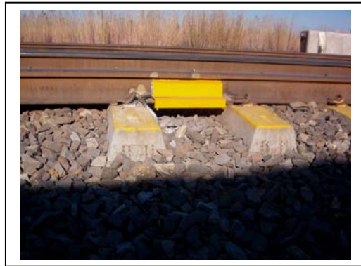
COVER PLATE OVER SENSORS
